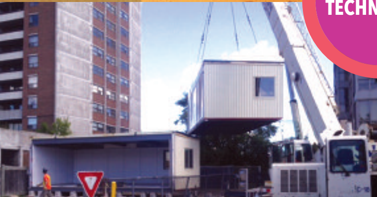
Above: The new Posluns portable is lowered into place
